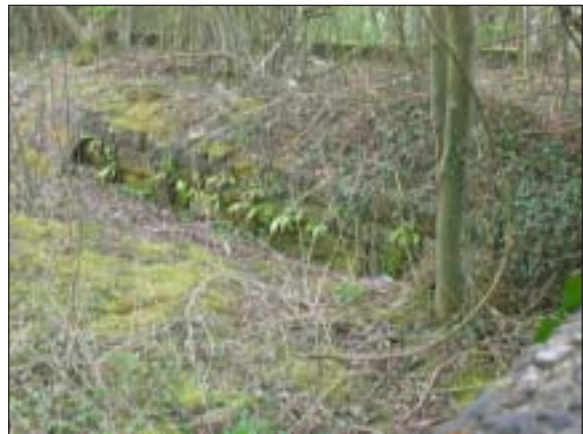
Remains of the bridge on the lane from Trevor to Cefn Mawr, demolished when the present Queen street was built in the 1960s. (SJ274425)
