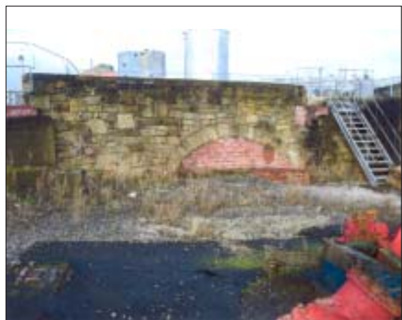
The bricked-up remains of the bridge within the Flexsys site. (SJ277426)
