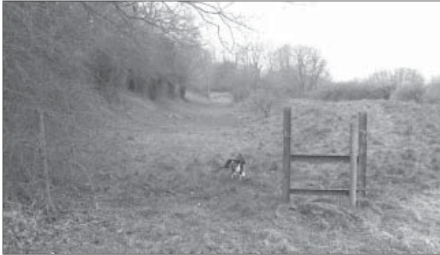
The profile of the canal, with a flat bottom to the channel, sides sloping at about 1:2, and a towpath on the downhill side. The method of construction whereby the left hand side of the channel is dug into the hillside and the material used to build up the towpath on the right as an embankment can be seen clearly. (SJ308555)
