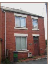
carefully pointed or rendered using lime mortar or render. The early Wrexham (Ruabon) bricks, were cleaned of their peeling paintwork to reveal their original character. Replacement bricks were sourced locally to re-instate the original proportions of the upper window.
