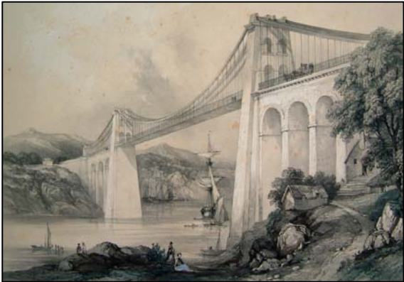
Menai Bridge of 1826, by Dibdin
